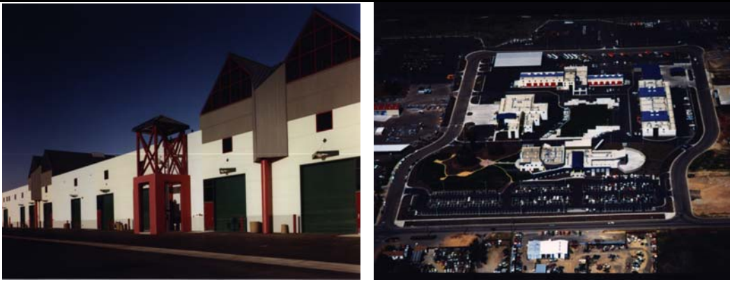
Figure 18. Examples of Tilt-Up Concrete Panel Building Type.
