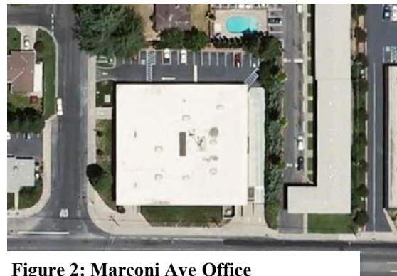
Figure 2: Marconi Ave Office
