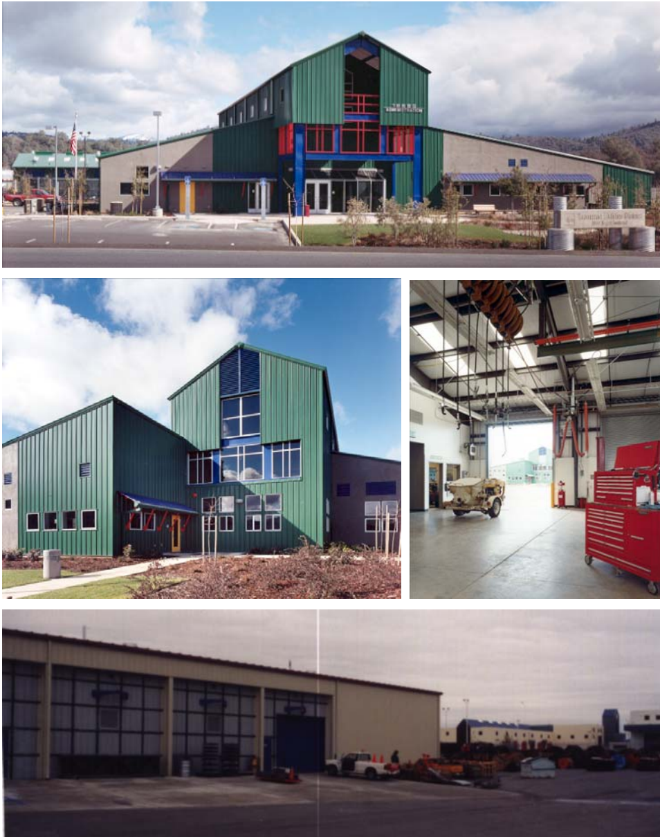
Figure 16. Examples of Pre-Engineered Metal Building Type.
